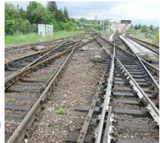
Water Orton Resignalling
