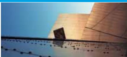
Right: Our steel was used in the Eden Project in Cornwall, UK.
