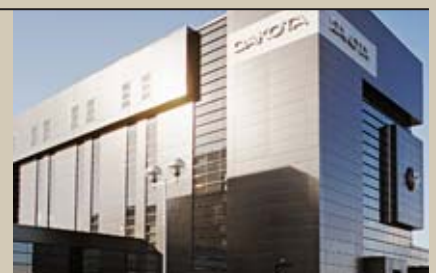
Right: The Dakota Hotel in Motherwell, Scotland, uses Colorcoat Prisma® pre-finished steel as part of the wall cladding.
