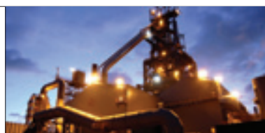
Blast furnace no. 5 at Port Talbot
