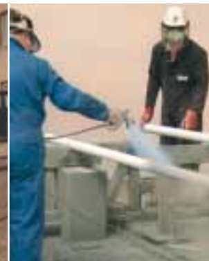
Application of sealant to aluminium sprayed columns.
