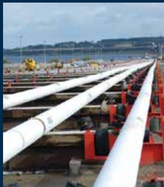
Coated pipe delivered to Evanton spoolbase ready for reeling onto CSO Apache lay vessel
