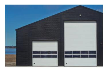
The entire building is made of steel and the construction took only 12 weeks. "On the steel rafters, which have a free span of 20 metres, we have mounted transverse steel battens, onto which we screwed the facades and roof. Construction was amazingly easy, and the installation went smoothly once we had the sheets and accessories on site," Bjarne Christensen says.
