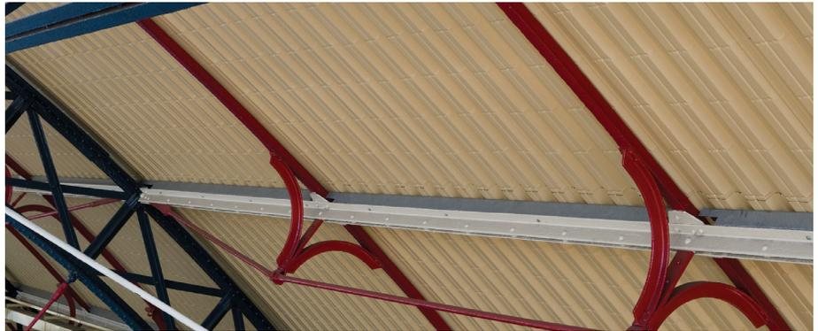
The replacement roof featured R46 profile in double-sided Colorcoat HPS200 Ultra®, with a Goosewing Grey finish on the external face and a Straw finish on the internal face. The R46 profile was selected by Network Rail due to its ability to span approximately 2.8m from purlin to purlin.
