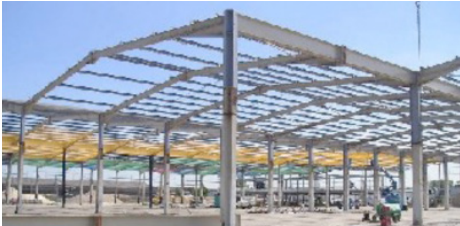
Figure 7. Refurbished portal frame ready for re-sheeting
