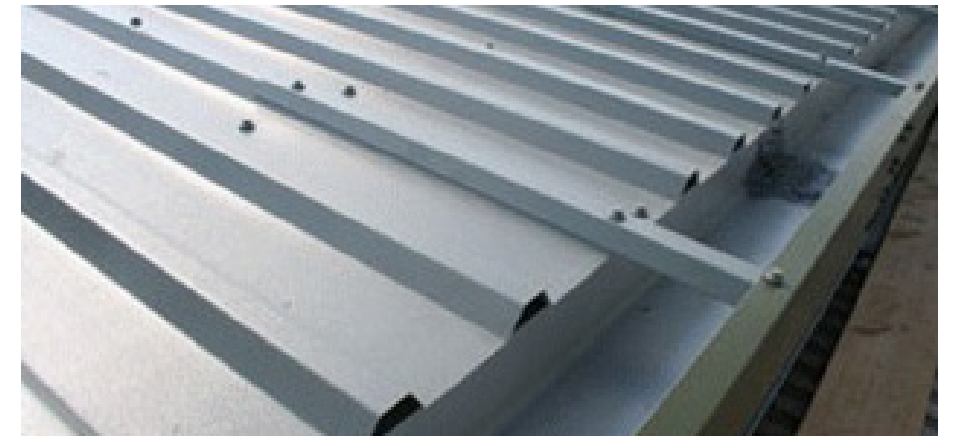
Figure 18. Roof after refurbishment showing pre-finished steel composite panel roof cladding
