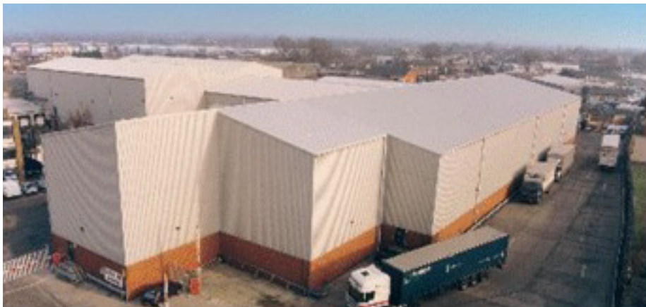
Figure 16. Refurbished building after pre-finished steel roof over cladding and the inclusion of improved insulation
