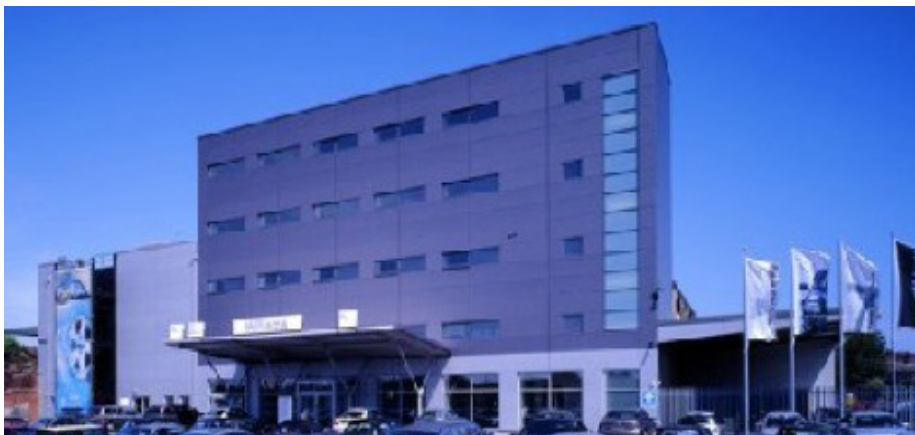
Figure 25. Building after pre-finished steel rainscreen over cladding system
