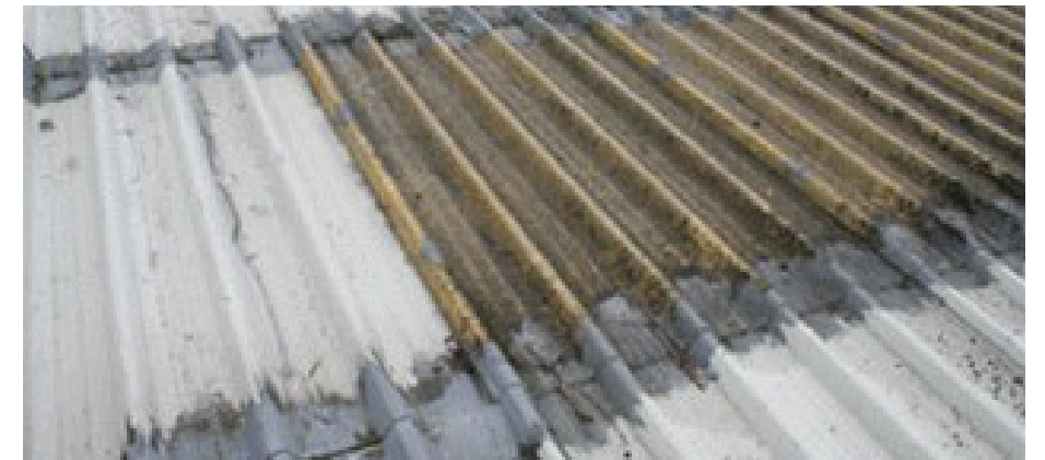
Figure 17. Before refurbishment showing failed roof cladding
