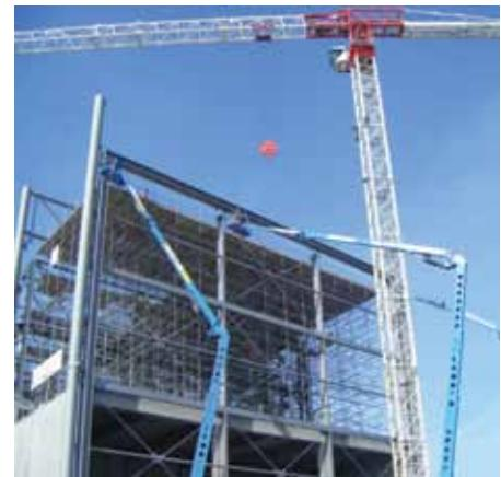
*"Use of circular hollow section allowed us to achieve the long spans required – it's strong but lightweight. The exposed steelwork on the EfW building is also visually effective. The sleekness of the trusses is particularly good."*
