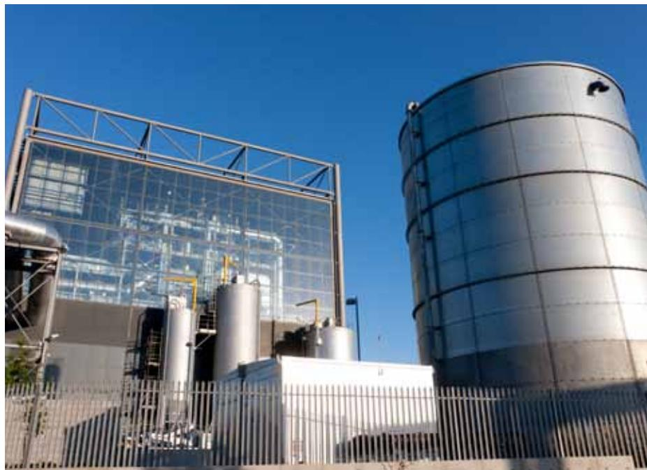
**"This large and complex steel structure really does showcase the benefits of Celsius® 355 Circular Hollow Section. It's far more efficient for spanning long lengths than open sections – cutting down on material requirement and fabrication. Because it's a hot-finished tube, there's no distortion when welding."**
