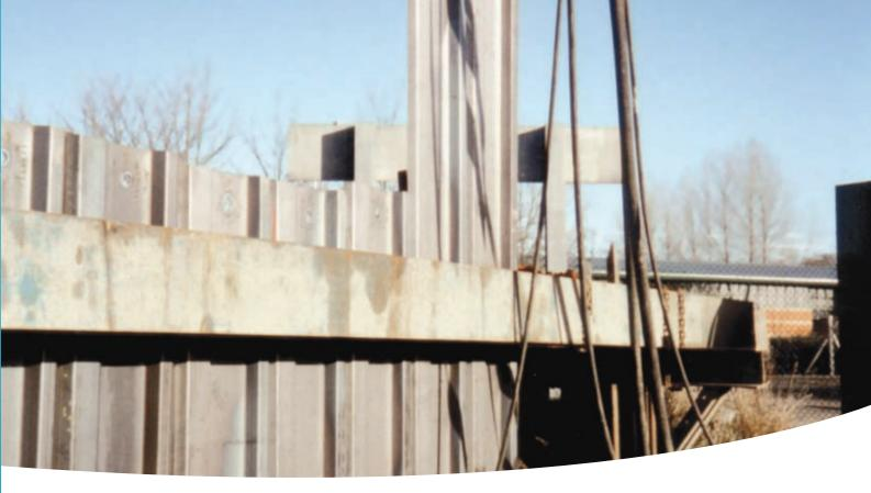
As a global manufacturer Tata Steel Construction Products are dedicated to the needs of the Construction sector. The strength, speed and flexibility afforded by trench sheeting makes it the ideal support solution. The durability and ease of extraction means that all Tata Steel Trench sheeting can be reused to encourage sustainable construction.
