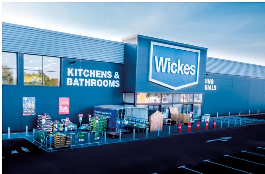
feature on a number of the Wickes Stores, ran across the top of the Trimapanel® on the front elevation acting as a separator between the two units. LP1000 liner panels were also used internally.
