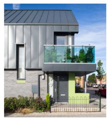
Catnic® Urban (formally Colorcoat Urban®) standing seam steel system, is a lightweight, strong and versatile alternative to traditional building materials that is seven times lighter than standard roof tiles.
