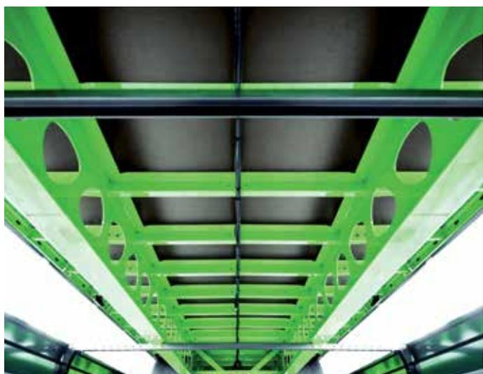
The only steel used is Ympress® S700MC from Tata Steel.
