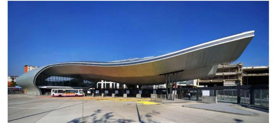
diameters of 193.7mm and 457mm. These were framed out with secondary and tertiary steel members to create the desired wave form. The undulating trusses, forming the 'backbone' of the canopies, vary in height off the ground. The canopies are clad in aluminium shingles to enhance the sense of movement.
