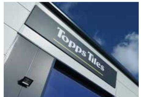
Although the Trimapanel® FTF (frame-to-frame) system can span up to eight metres, in the case of the Solent retail units the maximum distance between stanchions was 7.5 metres with some sections at six metres in length.
