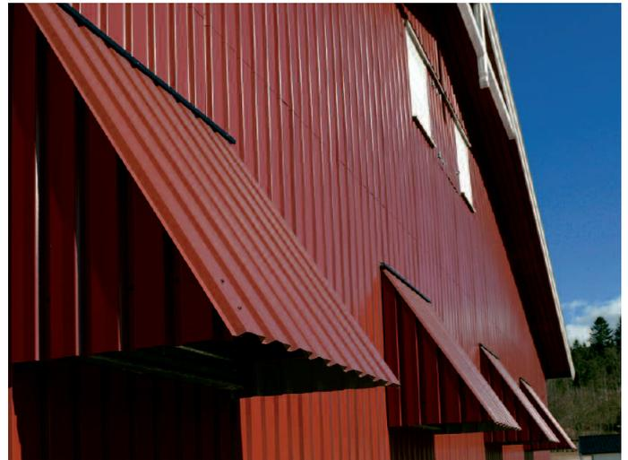
"The gable has four large exhaust ventilators concealed by hoods in the facing sheet. Aesthetically, this helps to break up the large wall surface. At the bottom of the facing sheets we have mounted a custom-made galvanized bracket. This prevents pests from entering and getting into the insulation."
