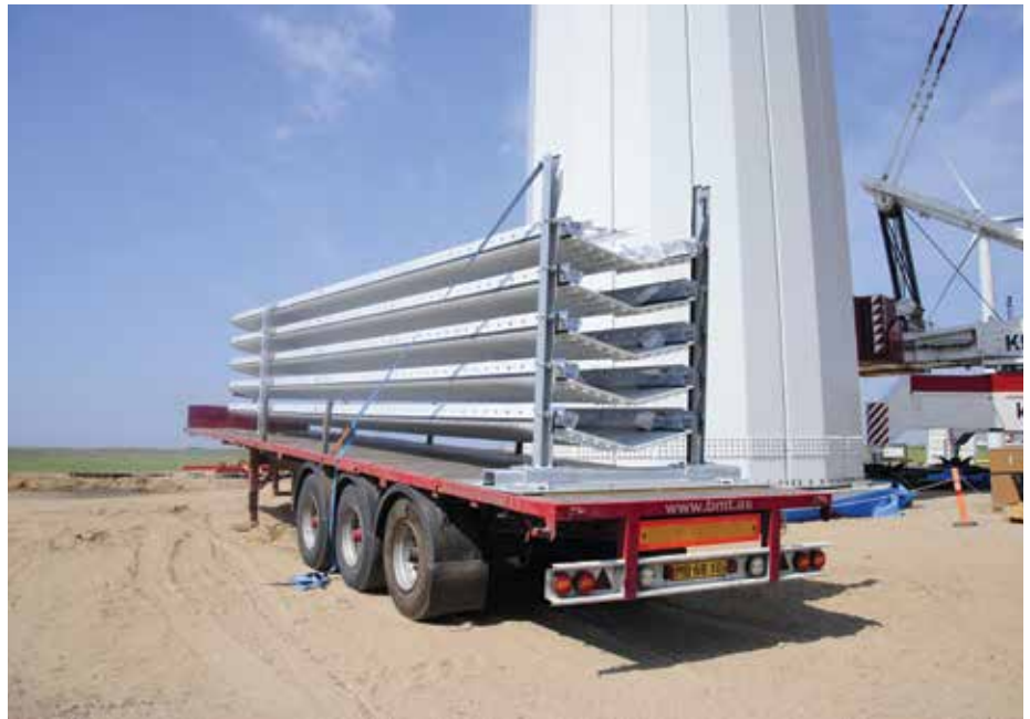
The new taller tower is uniquely bolted together on site.
